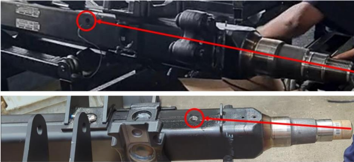
Figure 2: Top- exit hole on beam located between two spring pads. Bottom- Exit hole located between spring pad and wheel end
